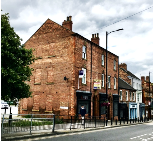
The side of the building, 2021. The blocked-up windows that once looked out onto Garden Street can be seen, and the street sign.
