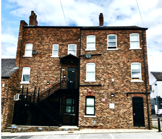
The rear of the building in 2021. On the right is part of the building that extended down Garden Street, and on the left the part that was John Smith's offices.
