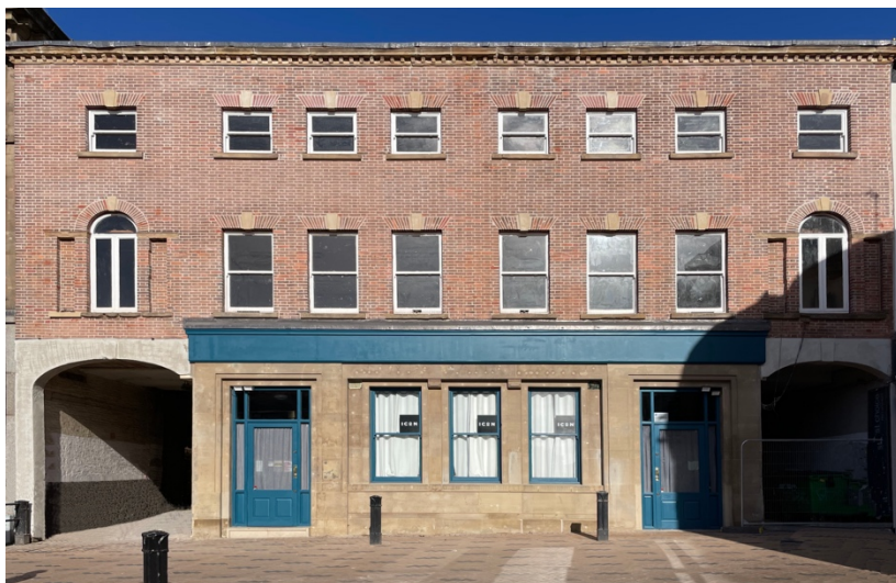
50 and 52 Westgate after renovations in 2022
