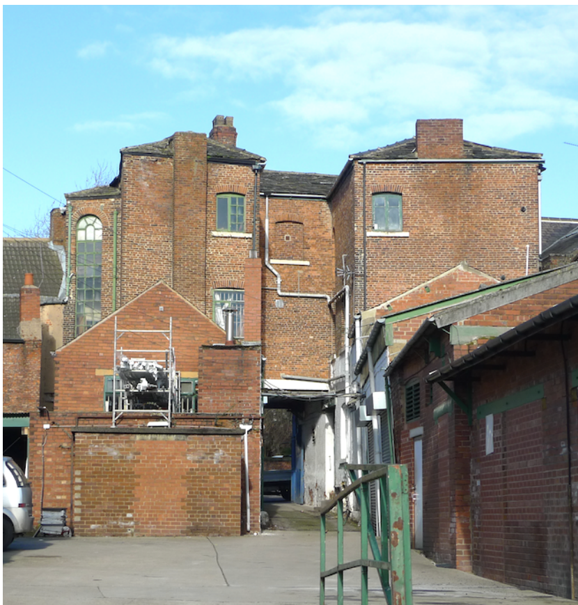
111 and 115 from the yard behind.
